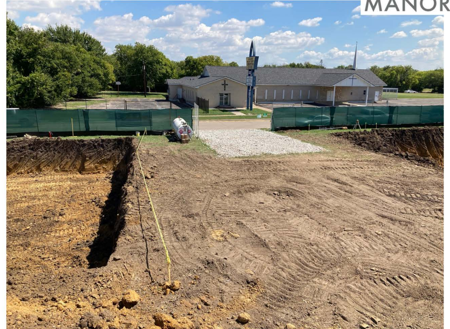
Site entrance with SWPP and bullnose rock for construction site entrance.
