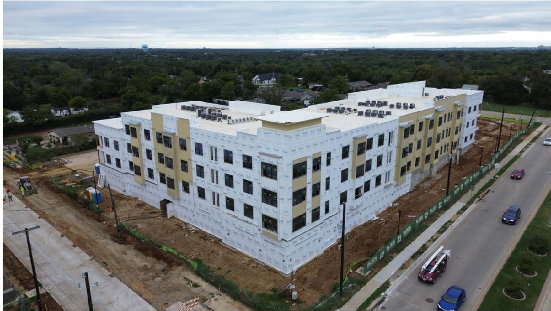
Aerial Photo: Building 1 facing southwest.
