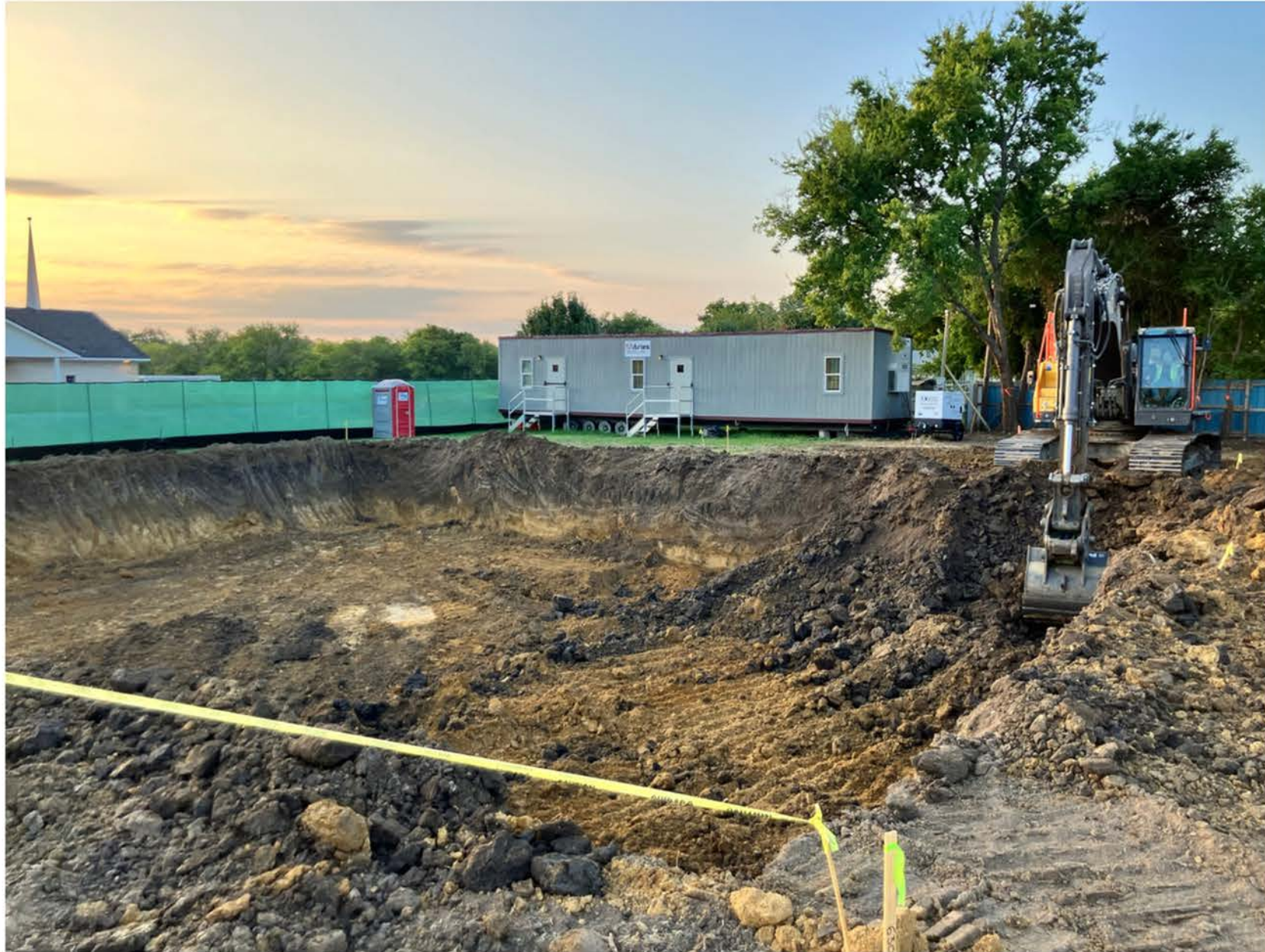
Excavation for building foundations.
