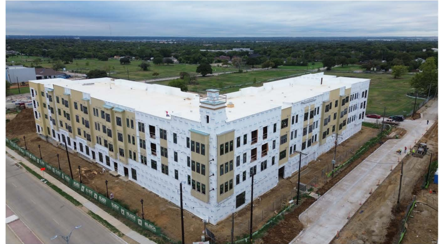
Aerial Photo: Building 2 facing southwest.
